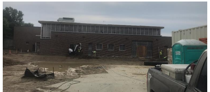
Clerestory window frames are installed
