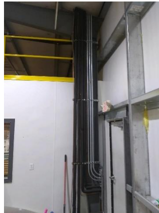
Refrigeration line and conduit for the air conditioners in the construction office
