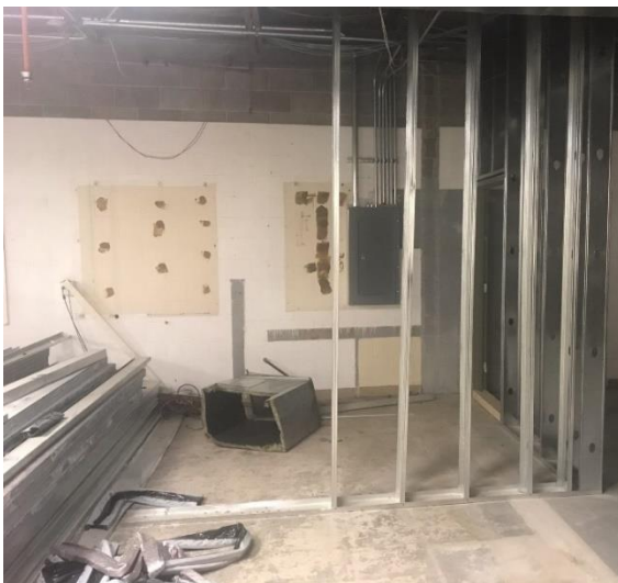
Framing around the new classroom area enclosing our new panel
