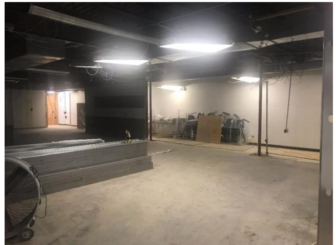
Demo complete in the hallway of remodel area
