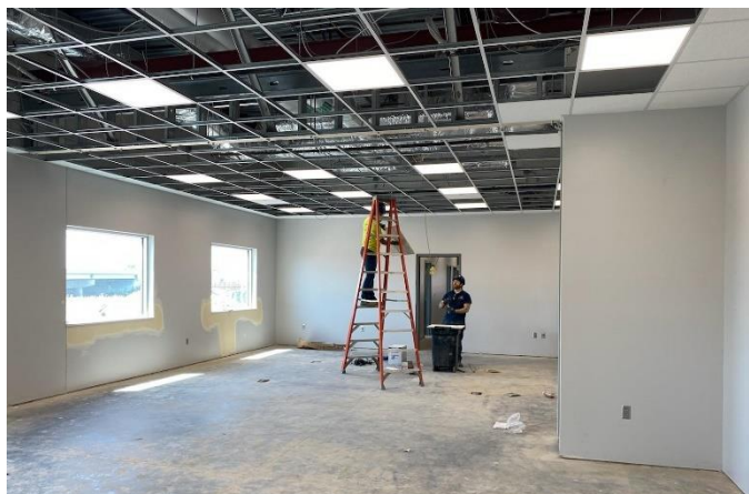
Nikki Prevail and Dakotah Whited working on some lighting controls in the conference room
