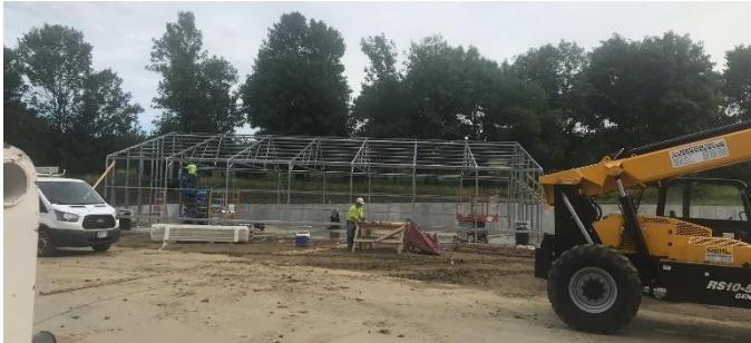
Greenhouse going up
